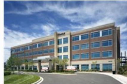
Depaul Medical Office Building Murfreesboro, TN
