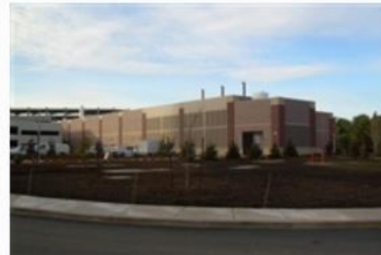
Sacred Heart Medical Center Central Utility Plant Springfield, OR
