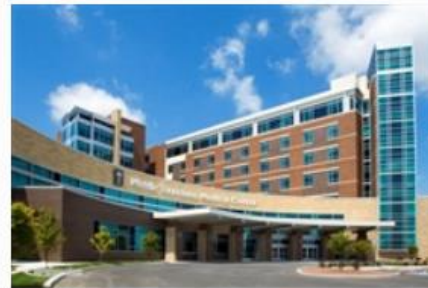
Middle Tennessee Medical Center Replacement Hospital Murfreesboro, TN
